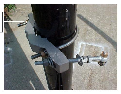
3. Fasten antenna and mount to the pole. Note that the pole mount rests on the shear stop U-bolt.
