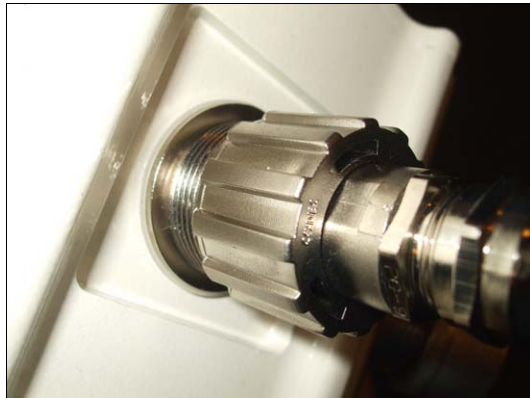
Figure 27: Complete Ethernet cap installation
